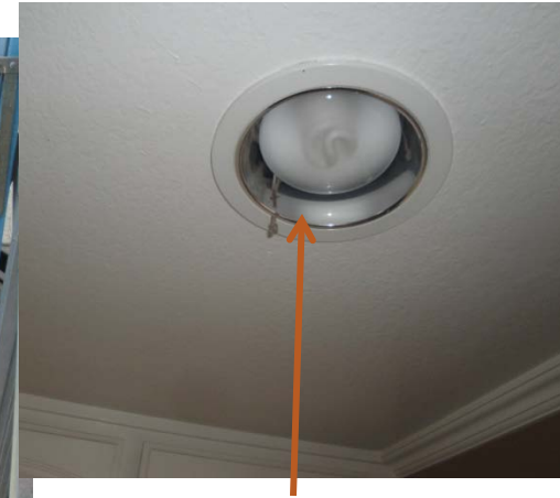
Dust/debris pulled through trim rings of most recessed lights. During blower door test.
